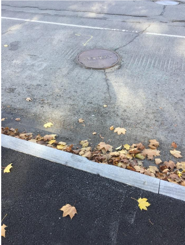
Sewer and Water
