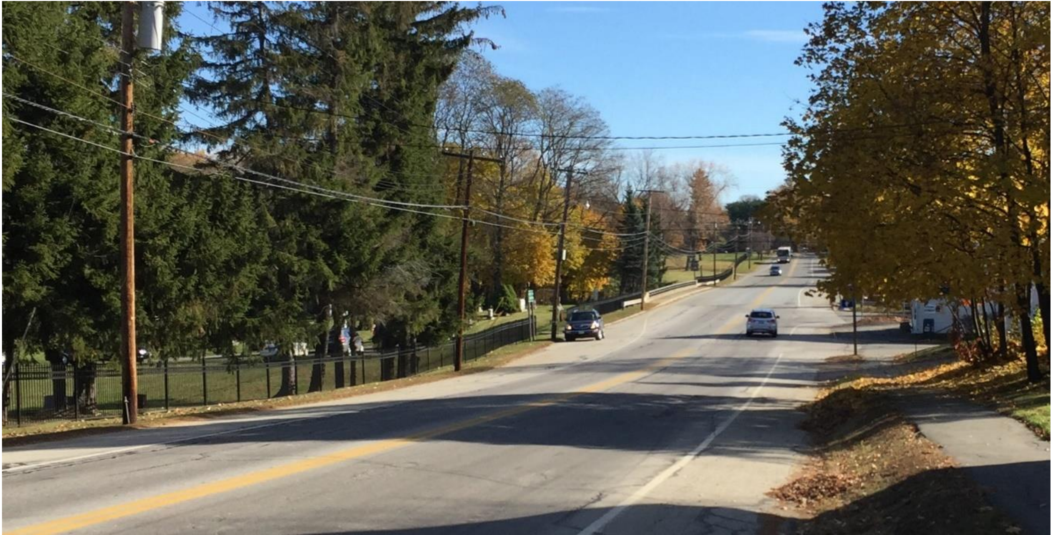
Ohio Street Looking East (Towards Bridge)
