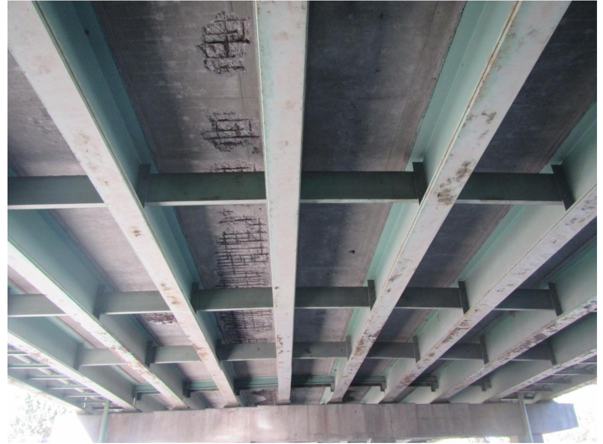
Underside of Deck over Travel Lanes
