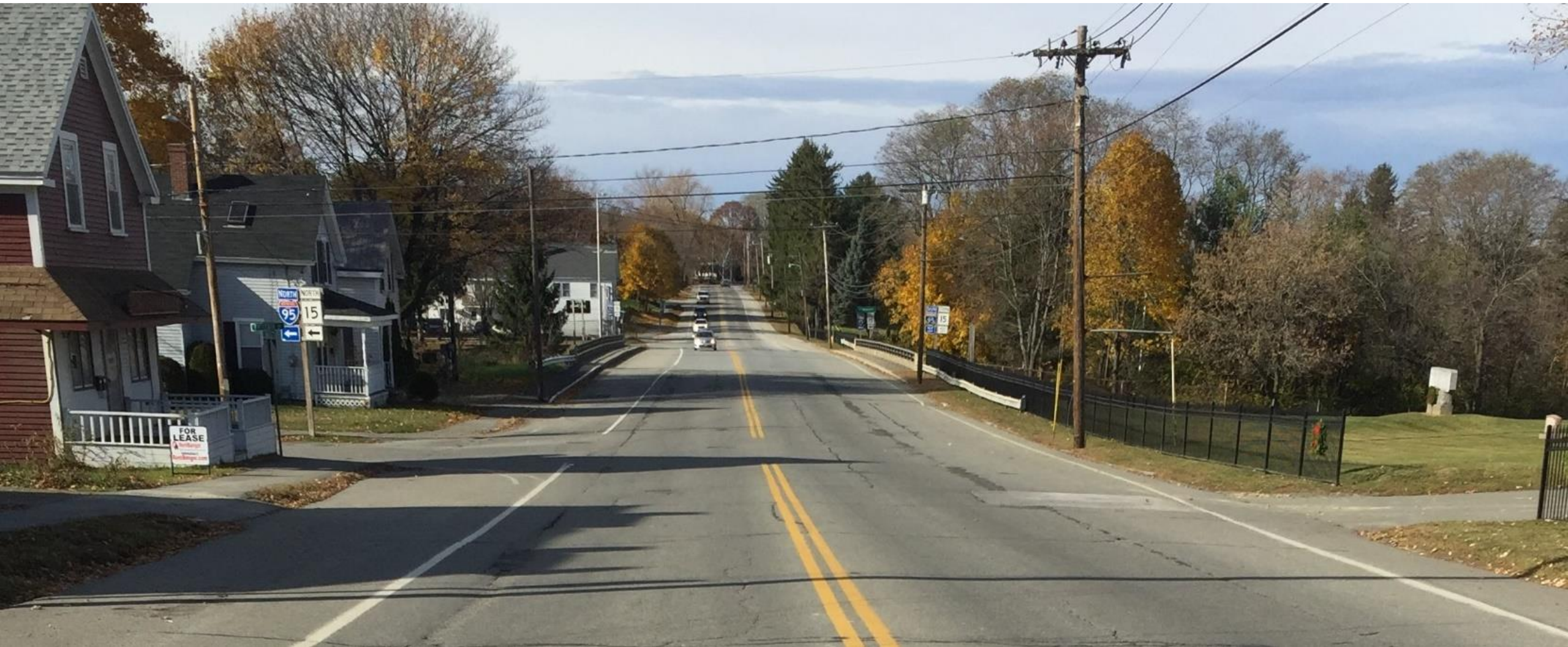
Ohio Street Looking West (Towards Bridge)
