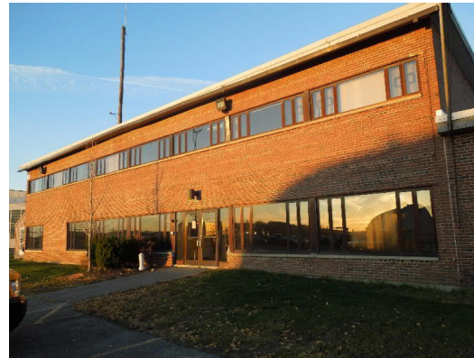
Figure 1. Building 96 Front Elevation
