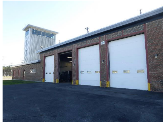
Figure 1. Building 253 GSE Shop
