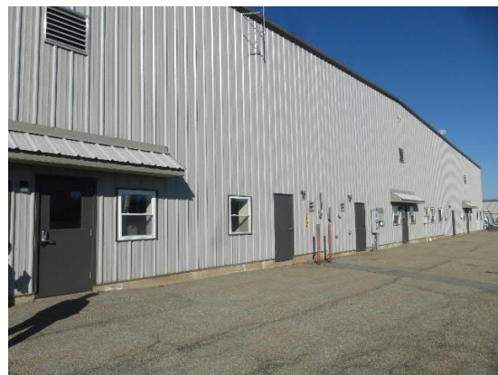
Figure 2. Building 123 Back Elevation
