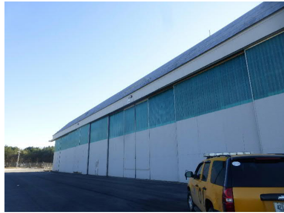
Figure 2. Building 252 Back Elevation
