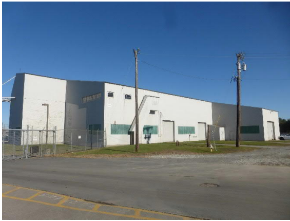
Figure 1. Building 252 Front Elevation
