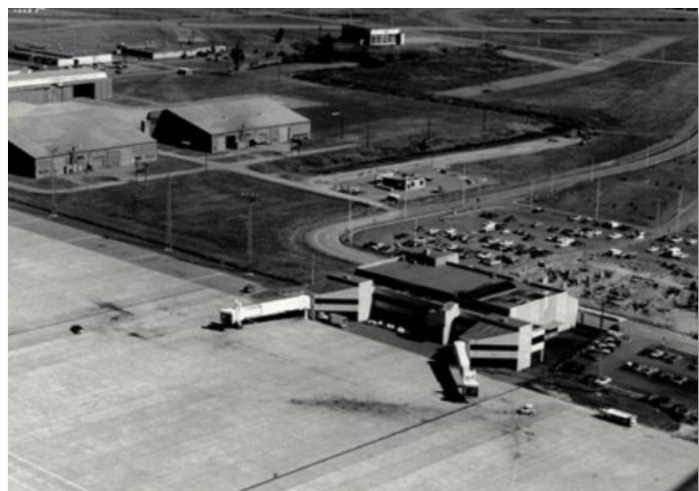
Figure 13 - Historic Photo: Domestic Terminal, circa 1972
