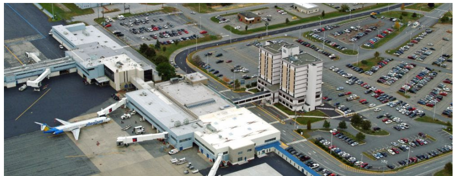
Figure 10 – Aerial of Existing Terminal Area Complex: International Pier (left) and Domestic Terminal (foreground) are not interconnected on the concourse's sterile side.
