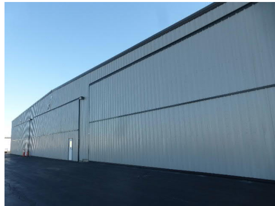
Figure 1. Building 123 Front Elevation
