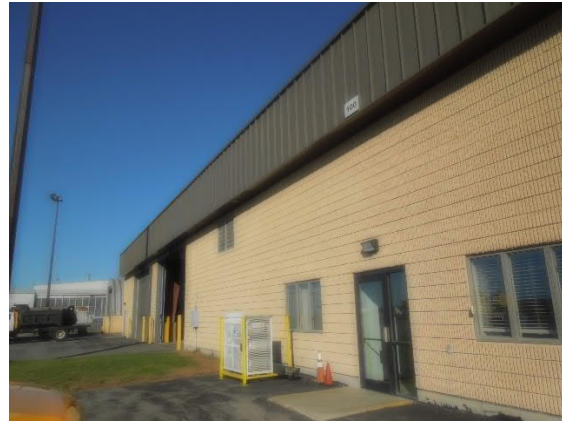
Figure 1. Building Front Elevation
