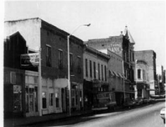
Figure 1. Inappropriate storefront alterations over the years—metal cladding, oversized signs and canopies—have detracted from the character of this historic district in Van Buren, Arkansas. A carefully considered rehabilitation plan for Main Street, including the removal of poorly designed signs, false fronts and the selection of an appropriate exterior paint color palette, serves to enhance the visual environment and preserves the district's sense of time and place. Photo above: Bob Dunn; Drawing: David Fets.
