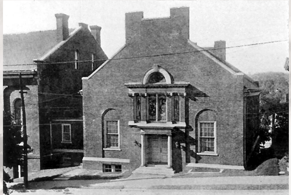
Renovated & Expanded Universalist Church
